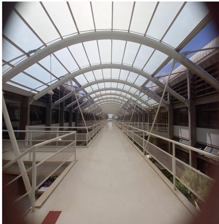
Figure 2: Structure of the Chemistry Building – IQ/UNB
