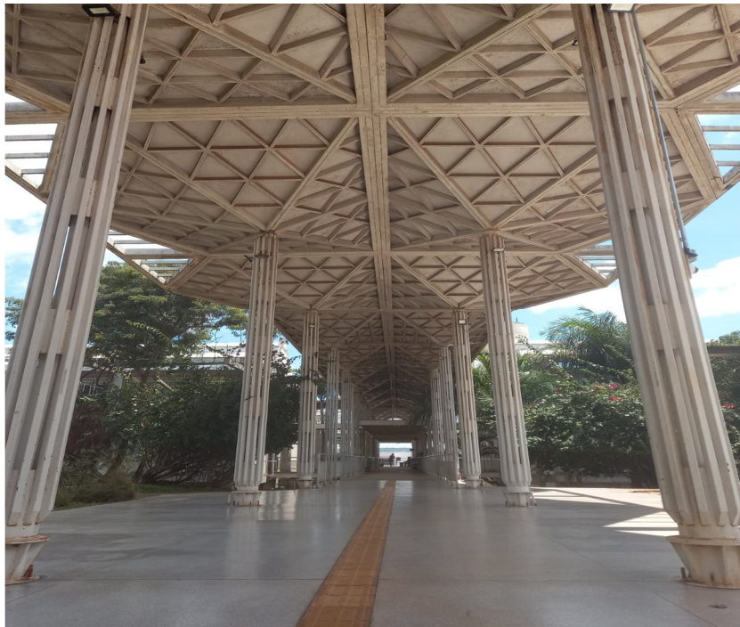
Figure 4: Structure of the Biology Building - UNB.
