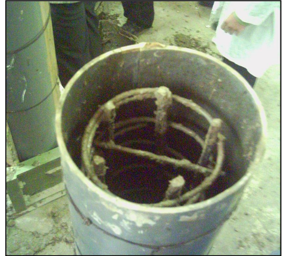
Fig. 2 column form with reinforcement
