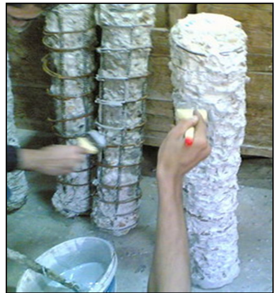
Fig. 4 Primer coated column surface
