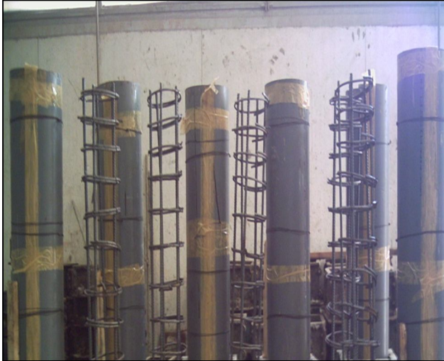
Fig. 1. Columns casting procedure
