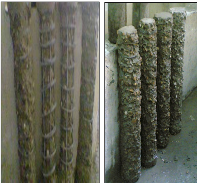
Fig. 3 Columns prepared to apply repairing
