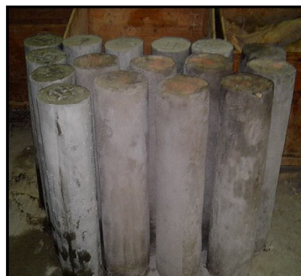
Fig. 6 Columns after repairing
